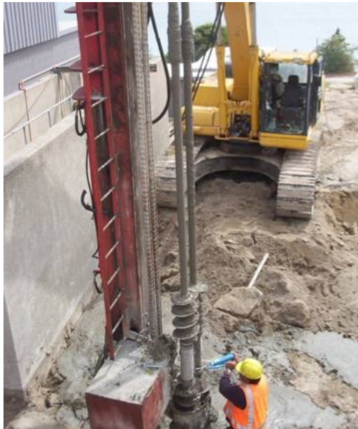
Figure 6: Tauranga WWTP site.
