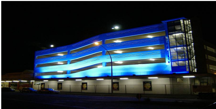
Figure 8: Knox Street Carpark, Hamilton - Inaugural use of DSM in building foundations.
