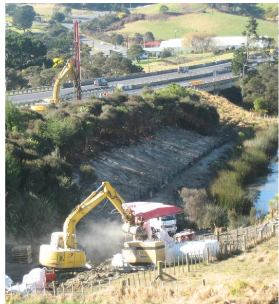
Figure 5: Installation of DSM columns at Okura.
